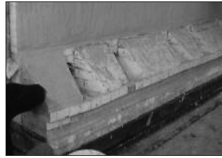
Application on ceramic fiber modules
